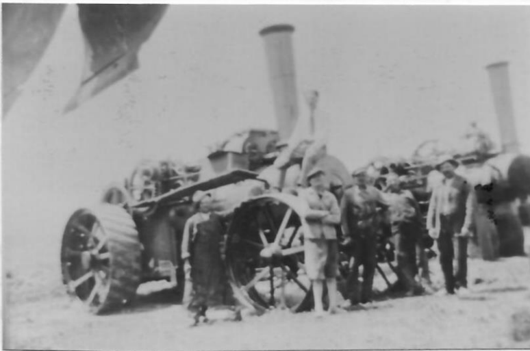
84. Steam engines for ploughing. Left top: shares of the tipped up plough shares
