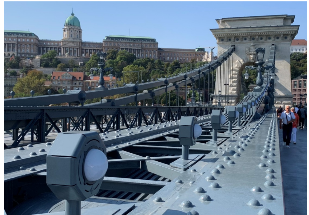
Up close & personal with the newly reopened and beautifully restored Chain Bridge, now restricted to pedestrians, public transport, taxis & bicycles. After a lengthy closure it felt like a real treat to walk over this one, which I duly did several times! Super paintwork, new LED lights (opposite, at night) which blend in fine. Adam Clark would be proud! Royal Palace and National Gallery on the hill in background.
