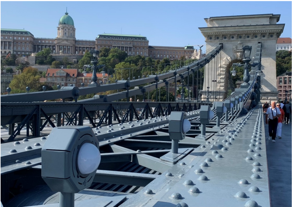
Up close & personal with the newly reopened and beautifully restored Chain Bridge, now restricted to pedestrians, public transport, taxis & bicycles. After a lengthy closure it felt like a real treat to walk over this one, which I duly did several times! Super paintwork, new LED lights (opposite, at night) which blend in fine. Adam Clark would be proud! Royal Palace and National Gallery on the hill in background.
